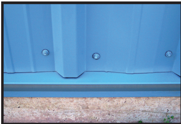
Example of a wall using McElroy's Base Trim.
