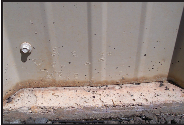
Contact with concrete can cause a wicking effect, resulting in premature corrosion.
