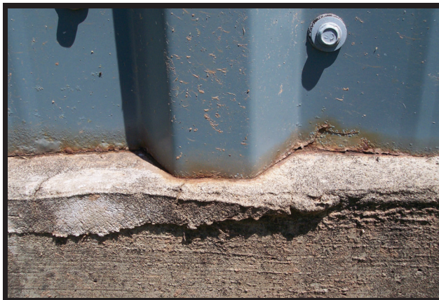
The flat areas of panels, as well as ribs, can all experience corrosion.
