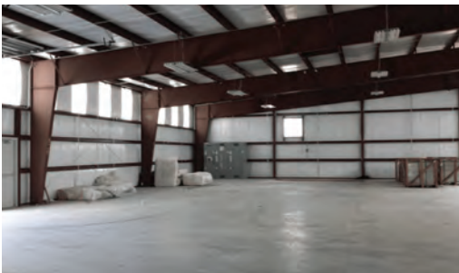
Traditional pre-engineered metal building interior featuring heavy duty welded framing members.
