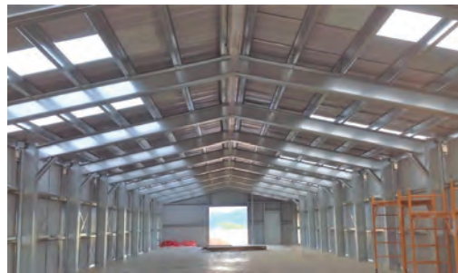
Pre-engineered cold-form metal building interior featuring light gauge roll formed framing members.
